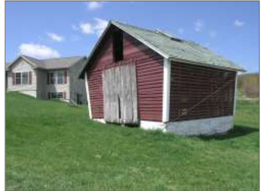
Exhibit 6-1. An example of a rural accessory building
