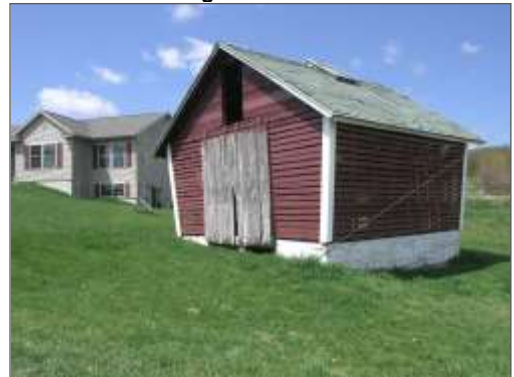
Exhibit 6-1. An example of a rural accessory building
